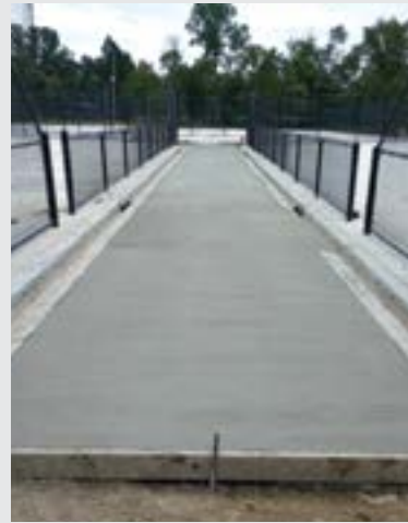
Holly Tennis Courts sidewalks
